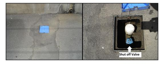
If required, the water supply to your house can be turned off by turning the shut off valve clockwise.
